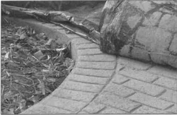
Example of Curved Area Edge Stamping at Sidewalk Intersection (Cleaning & Sealing not yet done)
