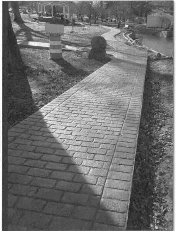
East of Run Sidewalk Looking South from Fairfax St (Section nearest camera is still wet (dark) from washing and sealant)
